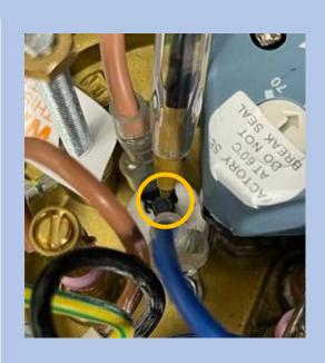
4. Thermostat gauge must then be turned down – twist gauge to 50 degrees. Screw the top cover back on and power EDDI back up to see if issue is resolved. If this issue continues, please contact the office directly.
